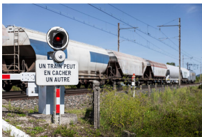
Railway Signal System
